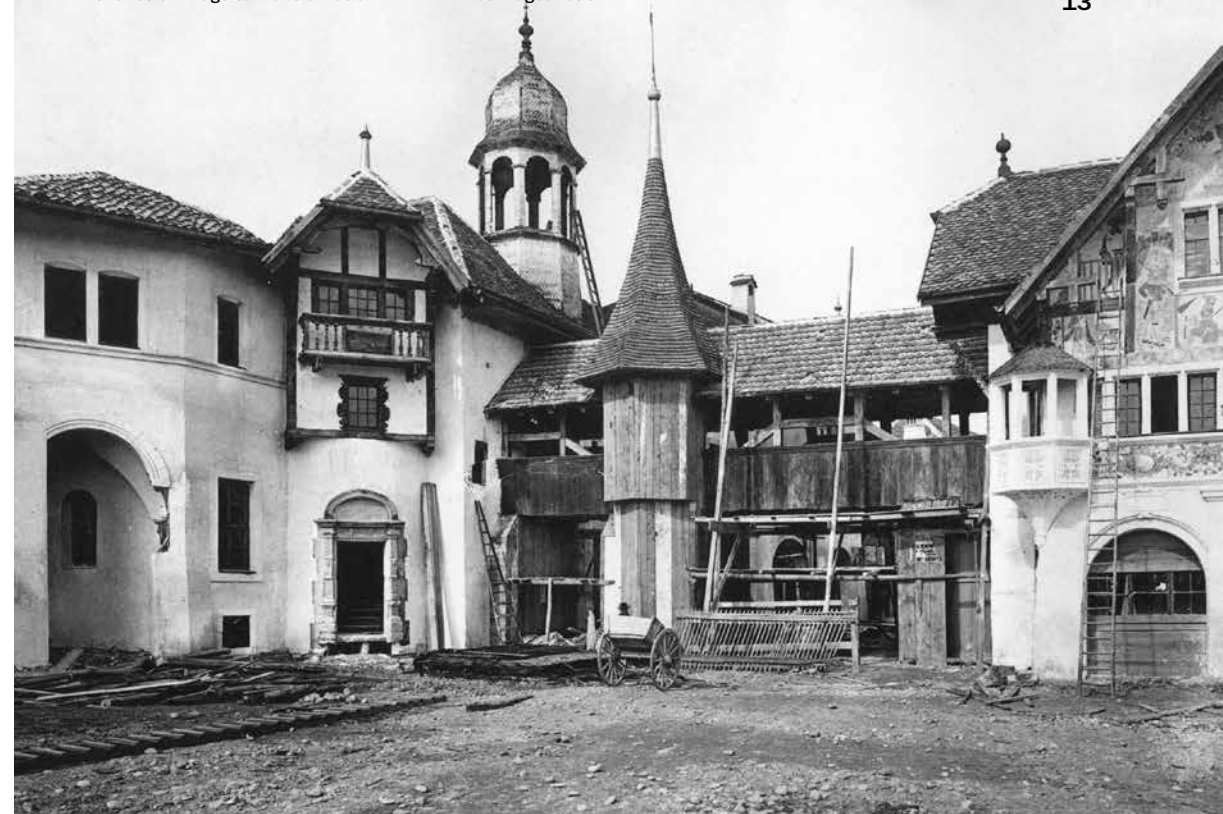
Paul Bouvier, Alois Brémond and Edmond Fatio, Village Suisse, Geneva, 1896: the entrance under construction/ Paul Bouvier, Alois Brémond en Edmond Fatio, Village Suisse, Genève, 1896: de bouw van de entree
