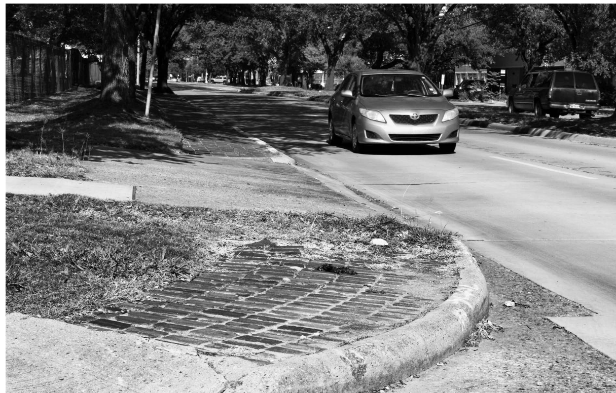
Brick sidewalk at Richmond Avenue/ Trottoir in baksteen op Richmond Avenue, Houston, 2022
