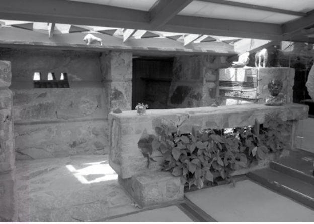
Taliesin West Studio, Arizona, Frank Lloyd Wright. Photo/foto Bruno Notteboom
