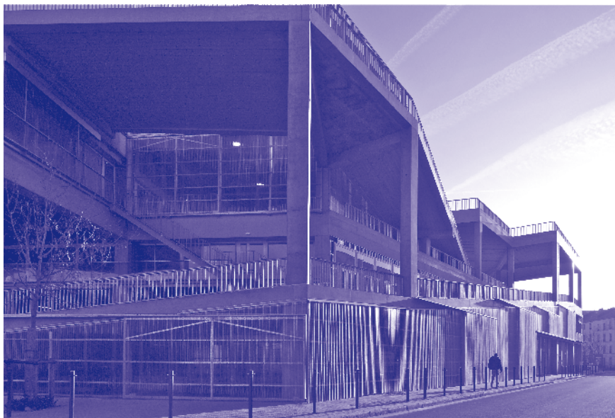
Lacaton & Vassal, Faculty of Architecture, Nantes, France, 2009
