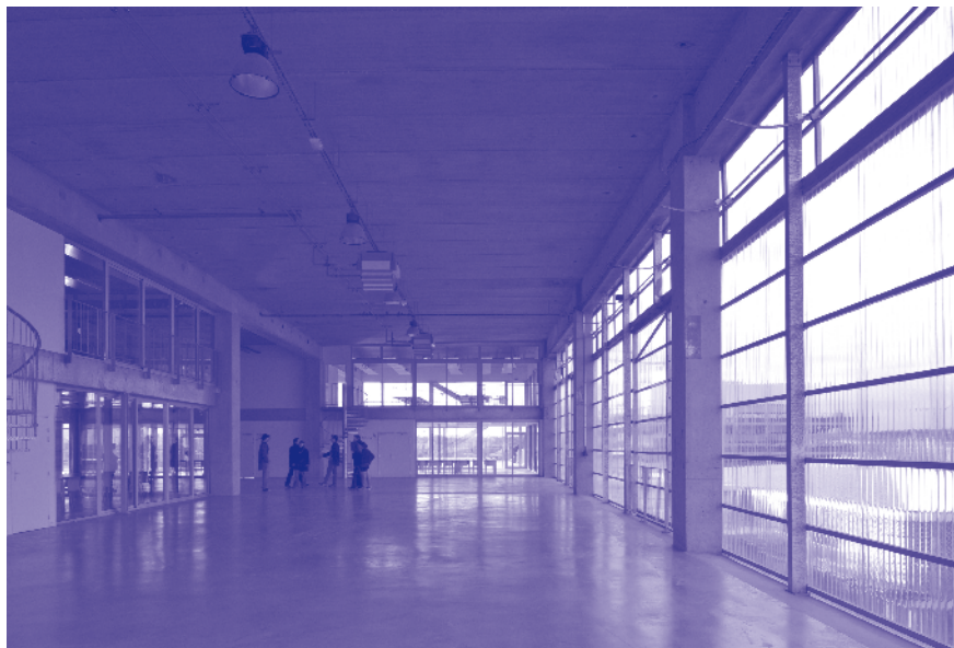
Lacaton & Vassal, Faculty of Architecture, Nantes, France, 2009
