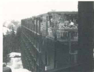
Arc 1800, roof terrace / dakterras
