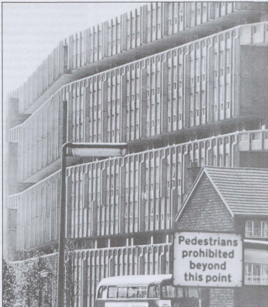
The Blackwall Tunnel South building's deck-side facade, seen foreshortened by telescopic lens across the Tunnel mouth
