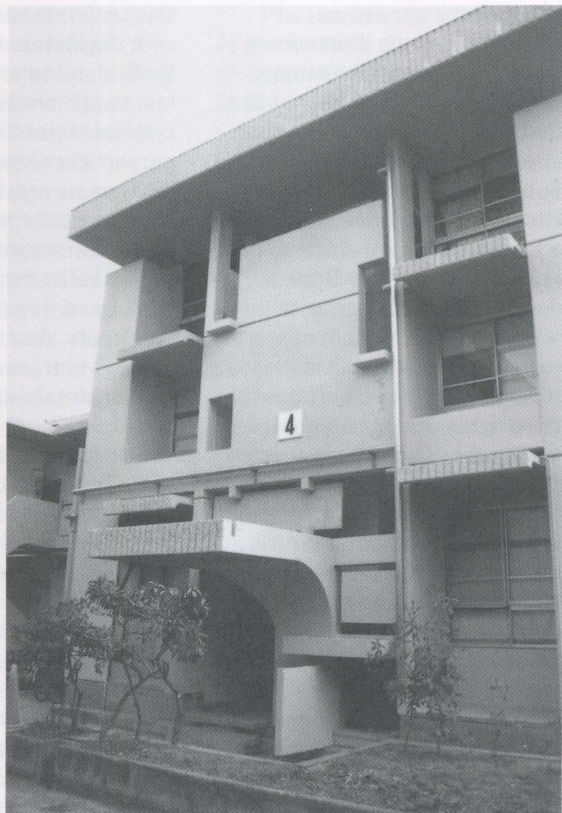
Gerenoeverde woningbouw / Renovated housing
